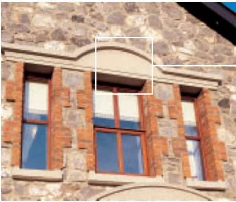
Elevation of window lintel
